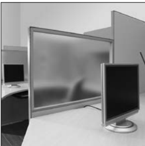
Partially glazed panels provide privacy and additional light
